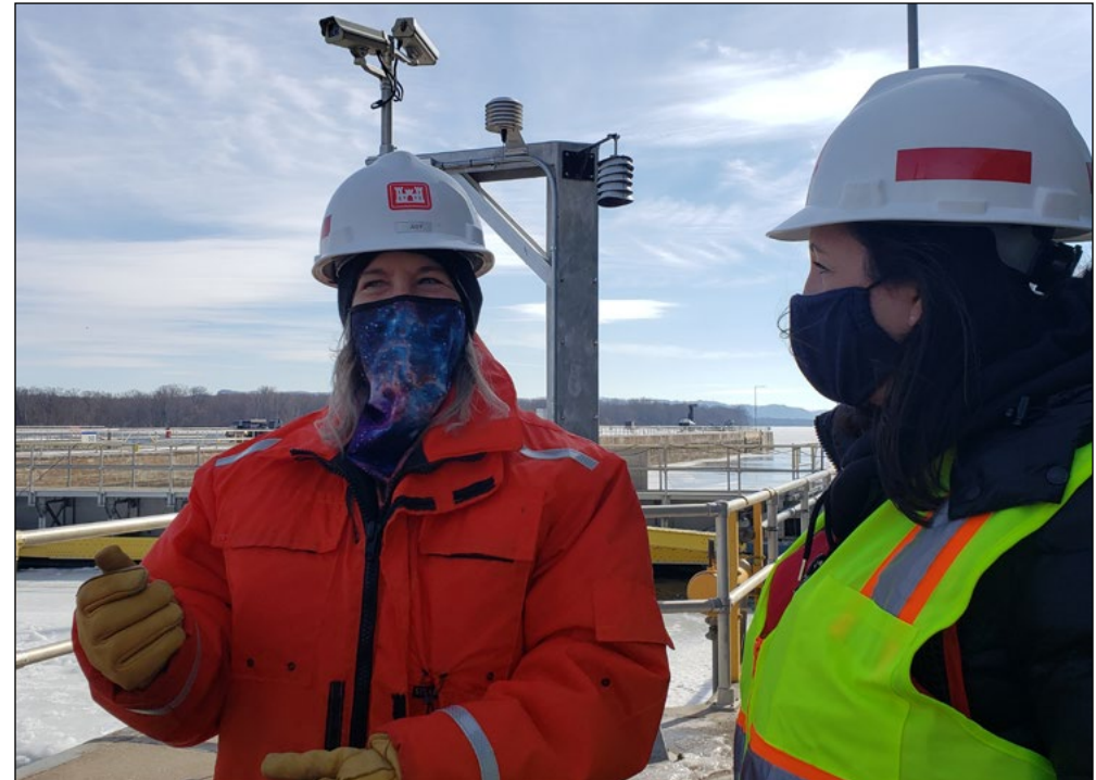
Judy Denzer, Lock and Dam 5 lockmaster, and Kim Warshaw, project manager, discuss the progress of the tow rail repair at Lock and Dam 5 near Minnesota City, Minnesota. USACE photo by Melanie Peterson
